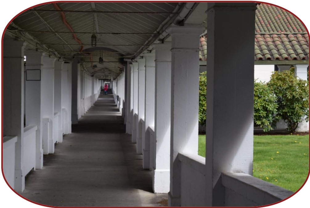
Photograph of a walkway at the Rainier School.
